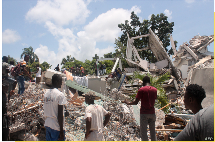
Building destroyed by the 7.2 magnitude earthquake, August 14, 2021, Ralph Tedy Erol
